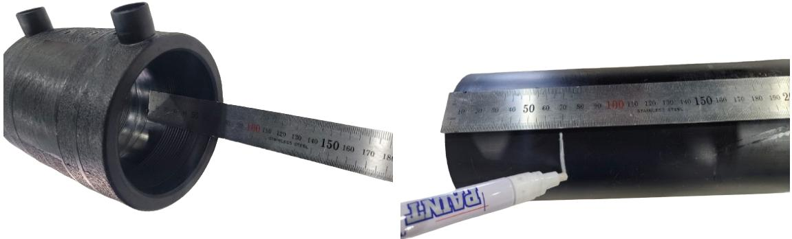
E. Scribe witness marks on the pipe surface or mark the area to be scraped or peeled in a criss-cross pattern.
