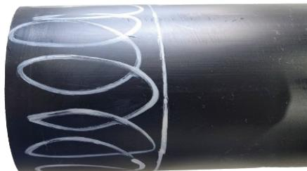
F. Remove the pipe surface layer by scraping or peeling to expose the clean virgin pipe material. Break shavings or remove them as needed to prevent them wrapping around the scraped or peeled pipe surface.
