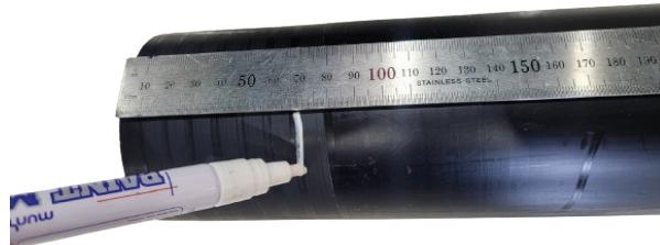
H. Insert the end of pipe into the coupling, up to the stab depth mark. Secure the pipe and fitting assembly to the alignment clamp.
