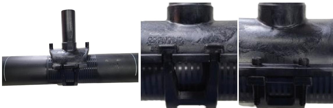
F. Connect the control box leads to the fitting, verify that the proper fusion time and voltage are displayed on the control box, and fuse the joint. Do not leave the fusion unattended.
