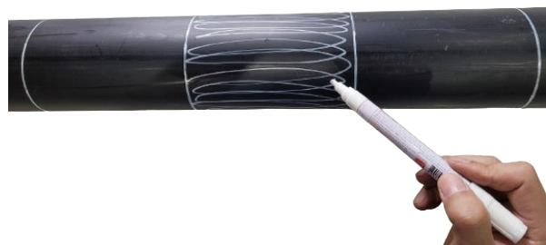
D. Remove the surface layer by scraping or peeling the pipe to expose the clean virgin pipe surface.
